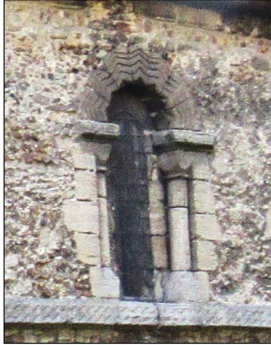
Figures 26 and 27: Photograph of the detail of the windows on the north elevation of the Cambridge Leper Chapel. Photograph at the left is the chancel window that was reportedly modified in the 15 th century and the window at the right is in the nave. It is nearly identical to the window on the southern elevation of the nave (Gjesfjeld 2019).
