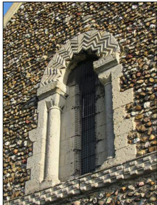
Figure 31: Photograph showing the detail of the window on the western elevation of the chapel. Stylistically, the window is the same as windows found on the nave; however, the crisp, clean lines associated with the carved Weldon stone serve as an indicator that the window was installed during the 19 th century rebuilding of the west wall by Gilbert (Gjesfjeld 2019).
