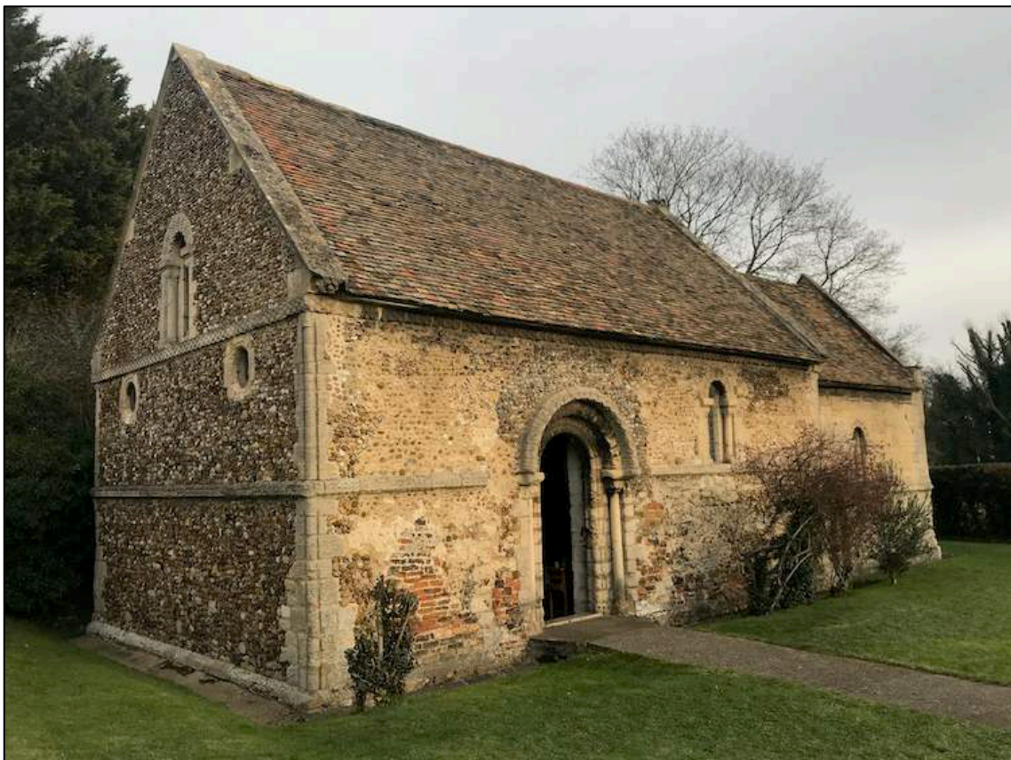
Figure 1: Photograph of the Cambridge Leper Chapel looking northeast showing existing conditions (Gjesfjeld 2019).
