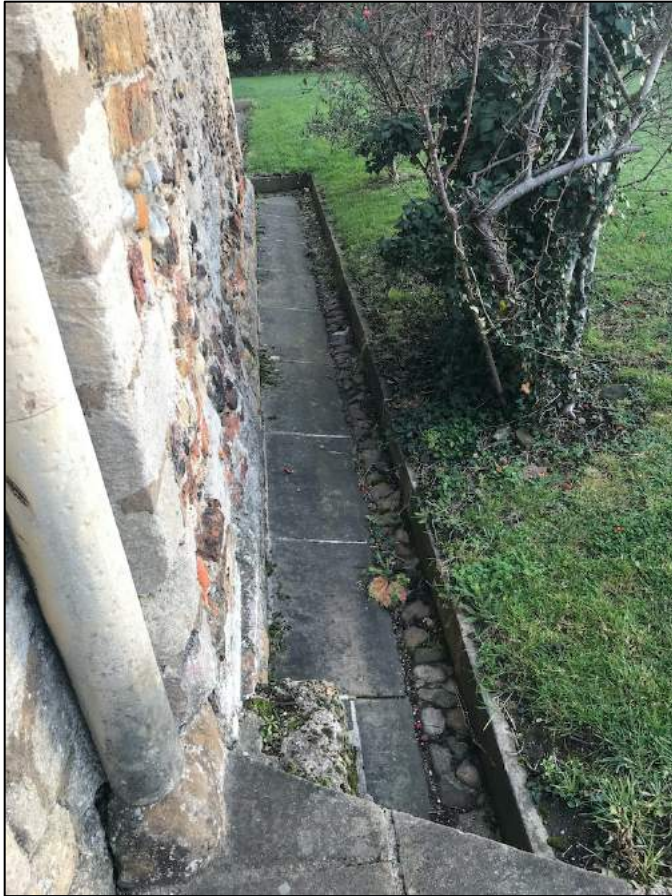
Figure 22: Photograph (above) looking east showing a drainage feature around the nave that was built to protect the building from dampness. The feature was installed at an unknown date, but further suggests modifications to the topography around the chapel (Gjesfjeld 2019).
