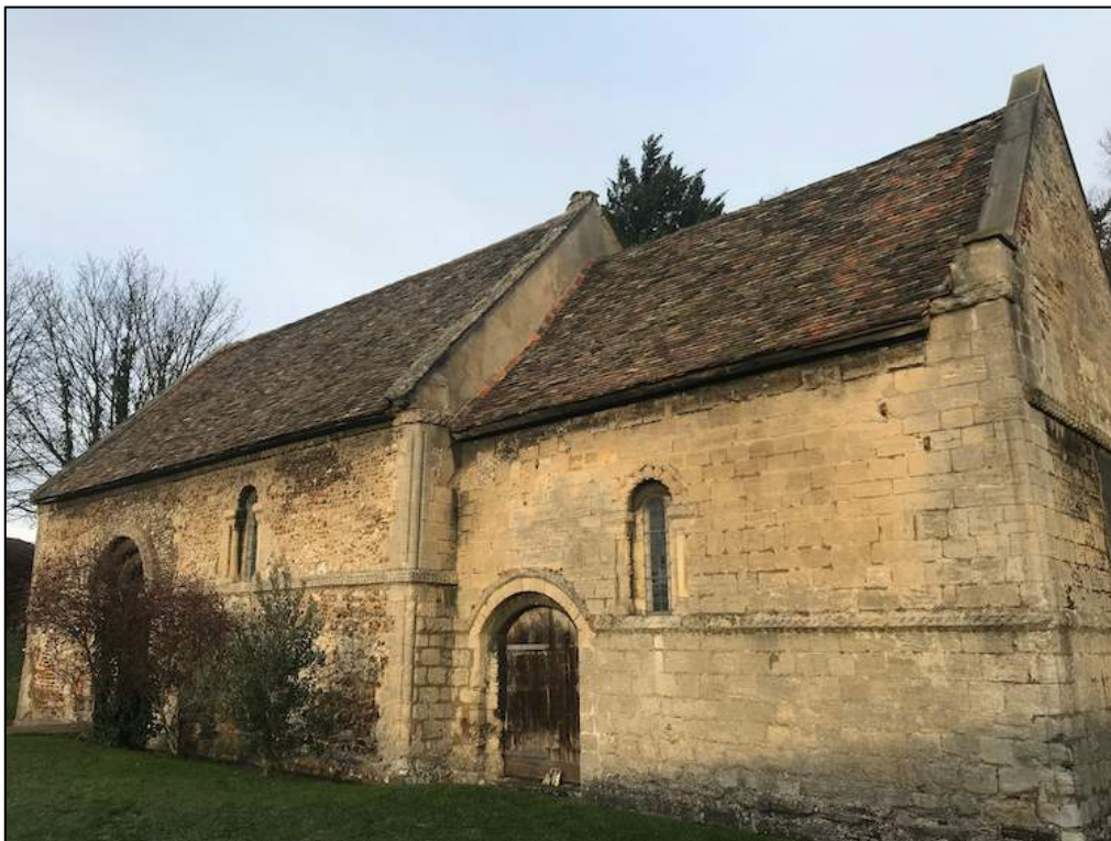
Figure 11: Photo of the Cambridge Leper Chapel looking northwest showing the primary façade of the building (Gjesfjeld 2019).
