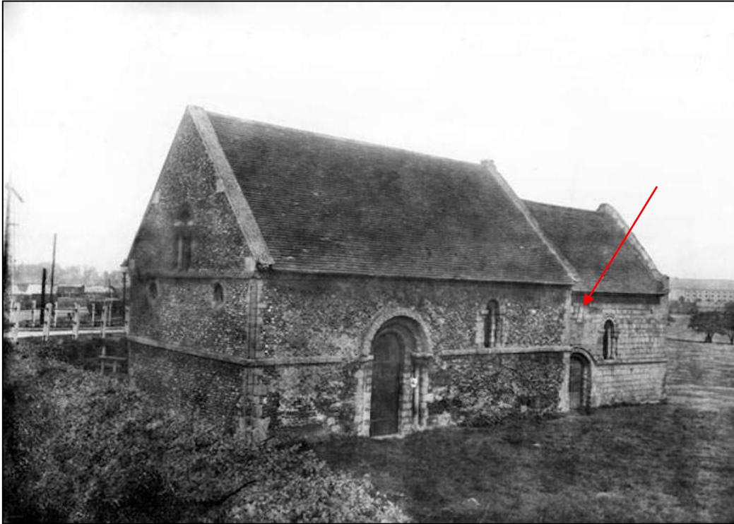
Figure 14: Photograph of the Cambridge Leper Chapel looking northeast, 1908. The photo was taken after installation of the Barnwell Junction station (left) in 1884 and before installation of the formal path leading to the front door in 1927. The red arrow shows the location of a former window with a noticeable repair (Historic England Archive ref: CC72/02035).
