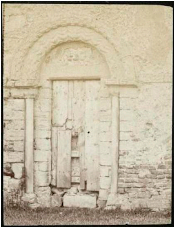
Figures 28 and 29: Historic photograph at left showing deteriorated condition of the door on the northern elevation of the chapel ca. 1875-1895 (Historic England Archive ref RBO01/05/OP22307). Photograph at the right shows the contemporary condition of the bricked-in door and its associated lintel and decorative features (Gjesfjeld 2019).
