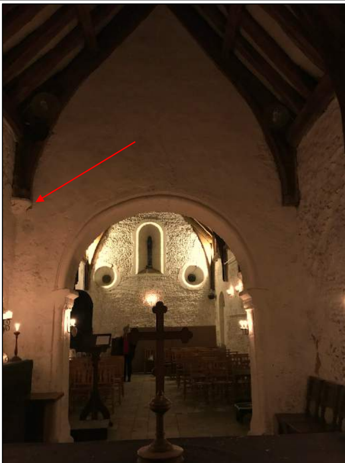
Figure 39: Photograph of the interior of the Cambridge Leper Chapel (above) looking toward the west wall that was reconstructed by Gilbert. This photograph illustrates the importance of the splayed window, which was designed to let more light into the chapel through the small windows (Gjesfjeld 2019).
