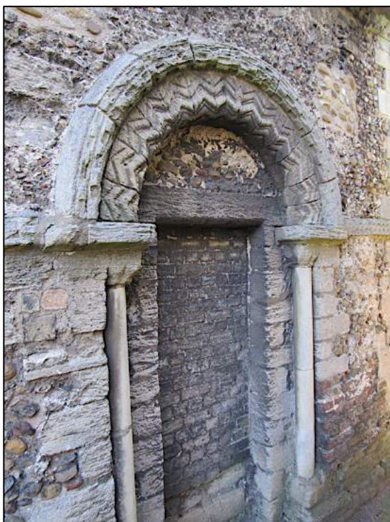
Figures 28 and 29: Historic photograph at left showing deteriorated condition of the door on the northern elevation of the chapel ca. 1875-1895 (Historic England Archive ref RBO01/05/OP22307). Photograph at the right shows the contemporary condition of the bricked-in door and its associated lintel and decorative features (Gjesfjeld 2019).
