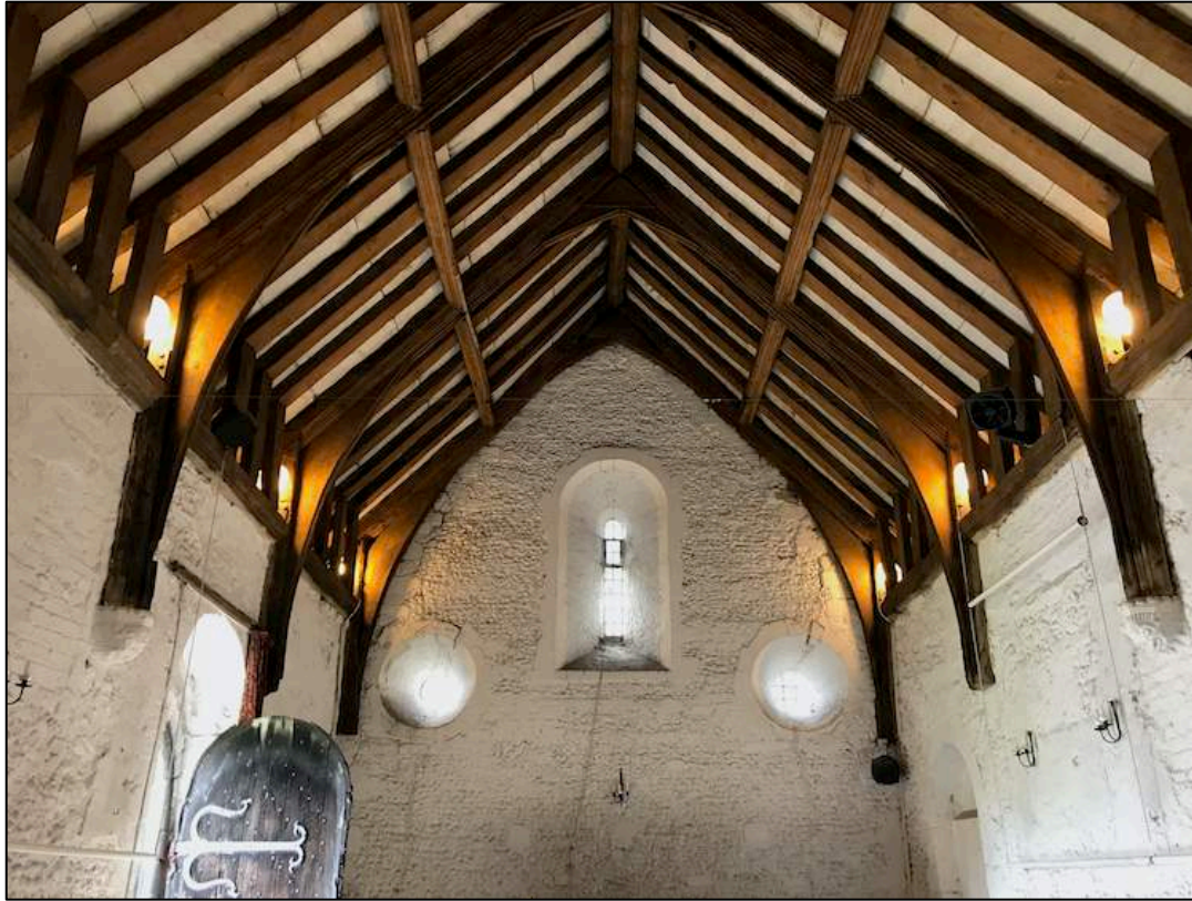
Figure 39: Photograph of the interior of the Cambridge Leper Chapel (above) looking toward the west wall that was reconstructed by Gilbert. This photograph illustrates the importance of the splayed window, which was designed to let more light into the chapel through the small windows (Gjesfjeld 2019).
