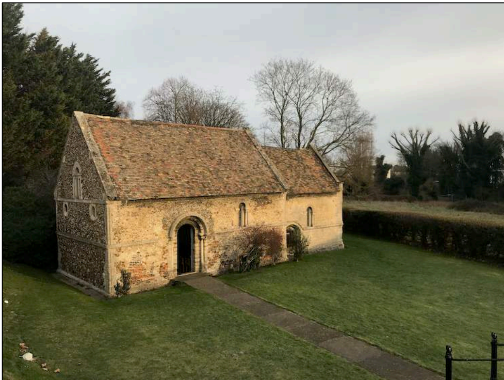
Figure 15: Photograph of the Cambridge Leper Chapel and its associated setting looking northeast toward the adjacent pasture that is separated from the building by a 20 th century hawthorn hedge (Gjesfjeld 2019).
