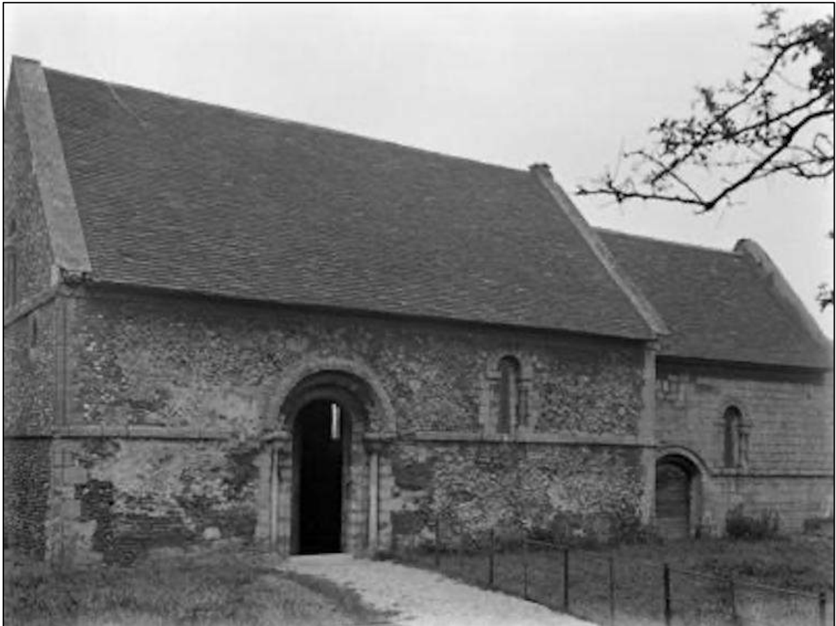
Figure 12: Photograph looking north showing the Cambridge Leper Chapel in June 1927. Note formalized path with handrail leading to the principal entrance of the building (Historic England Archive ref CC001431).
