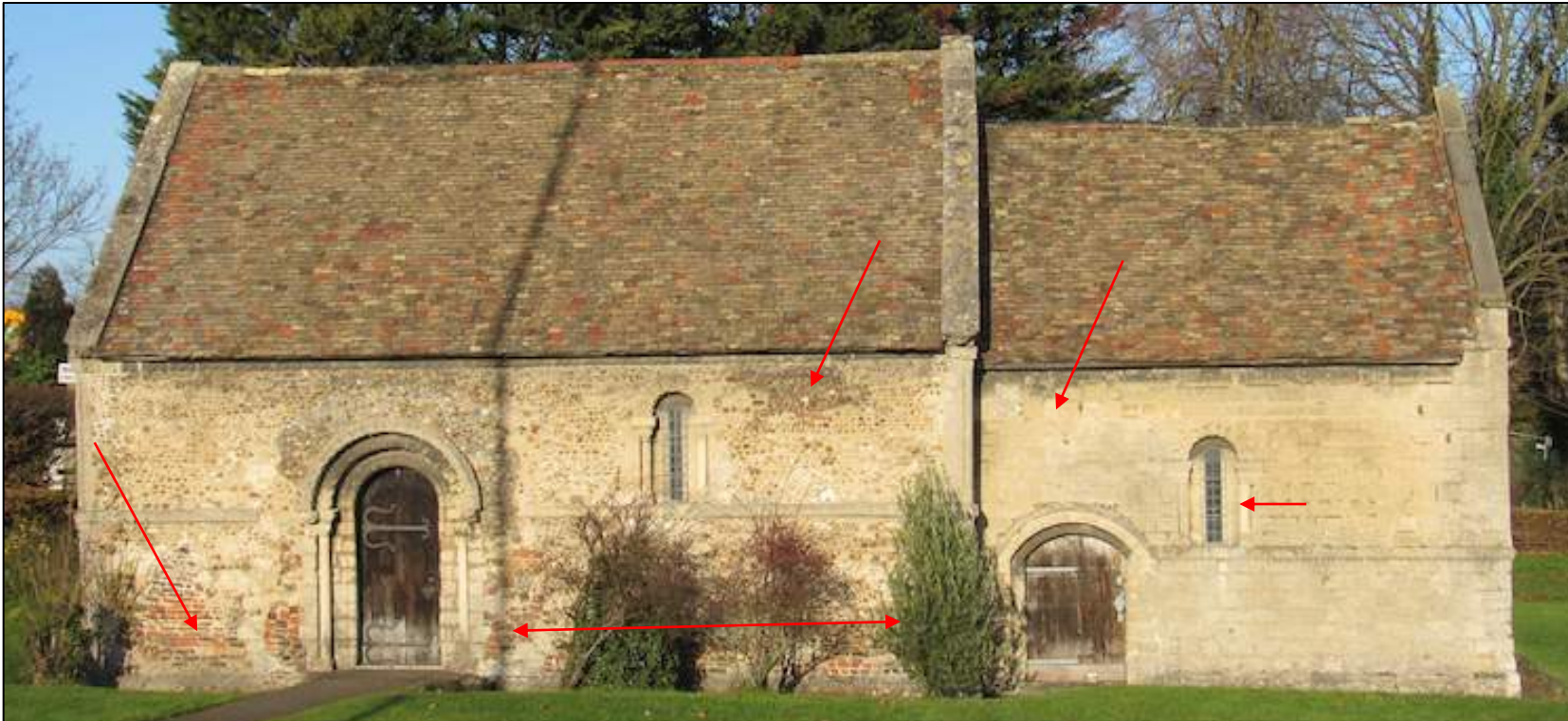
Figure 16: Photo of the Cambridge Leper Chapel looking northwest showing the nave (left) and the chancel (right). The red arrows at the far left and centre bottom shows a patchwork of materials including multiple shapes and sizes of bricks that were used to repair the nave under the string course. The two diagonal red arrows near the roofline show the approximate location of former windows noted in the 1725 drawing and Cotman's 1818 etching. The diagonal arrow in the nave illustrates a visible change in patina, while it is more difficult to see the former location of the window in the chancel. Generally, this side of the chancel shows the most refined finishing techniques, while change through time is more obvious on the other elevations. The arrow at the right in the chancel shows a replacement shaft near the window (Gjesfjeld 2019).
