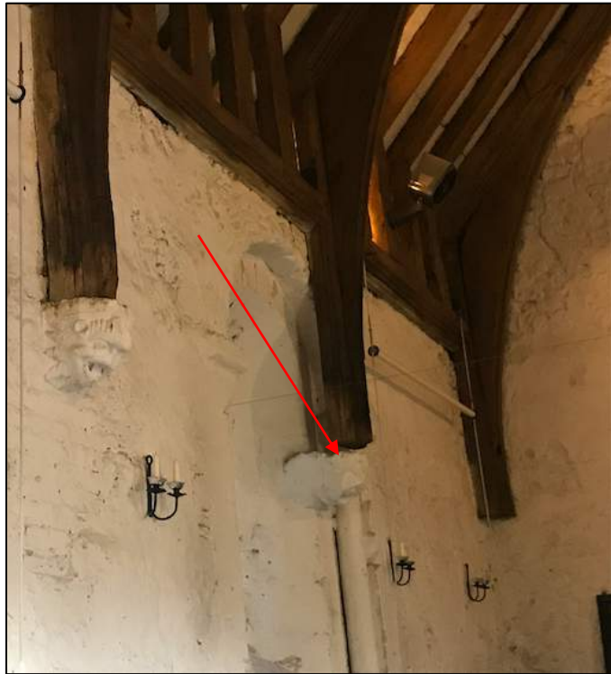
Figures 35, 36, 37 and 38: Photograph at the top left shows the interior of the Cambridge Leper Chapel and detail of the chancel arch. The red arrow points to the north wall of the chancel where there is evidence of fabric decay due to the application of masonry paint on the walls, which has trapped moisture (Gjesfjeld 2019). The red arrow in the photograph at top right shows 19 th century modifications made to the window opening in the chancel (Gjesfjeld 2019). The photograph at the bottom left shows the door on the northern wall of the nave that is blocked (Gjesfjeld 2019). The photograph on the bottom right shows the wall plate and associated timber posts in the nave. The posts conflict with the arched window openings and there is a gap between the corbel and the bottom of the post (Gjesfjeld 2019).
